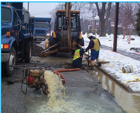
Water mains are more likely to break when temperatures dip below freezing. Waterworks crews are ready to respond 24/7.
