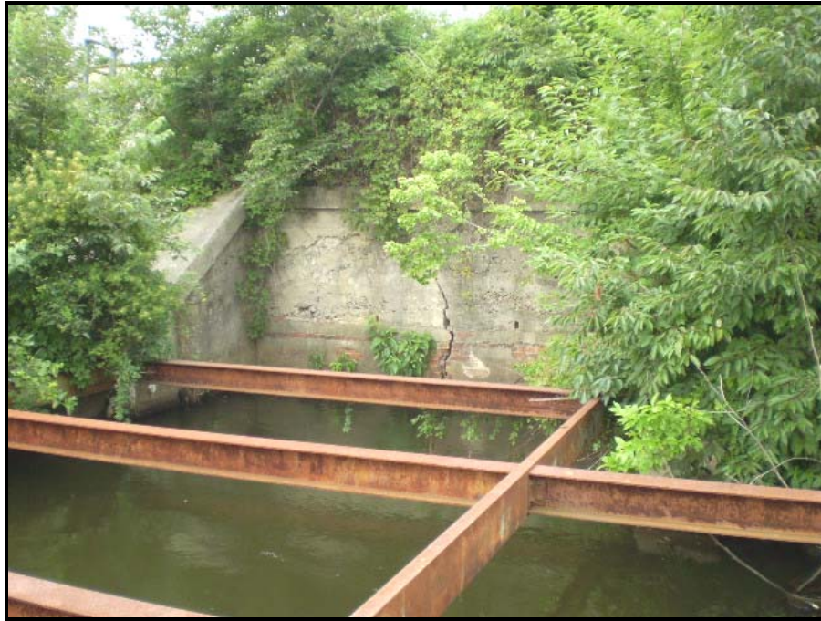
Photo 1 North (Upstream) Headwall
