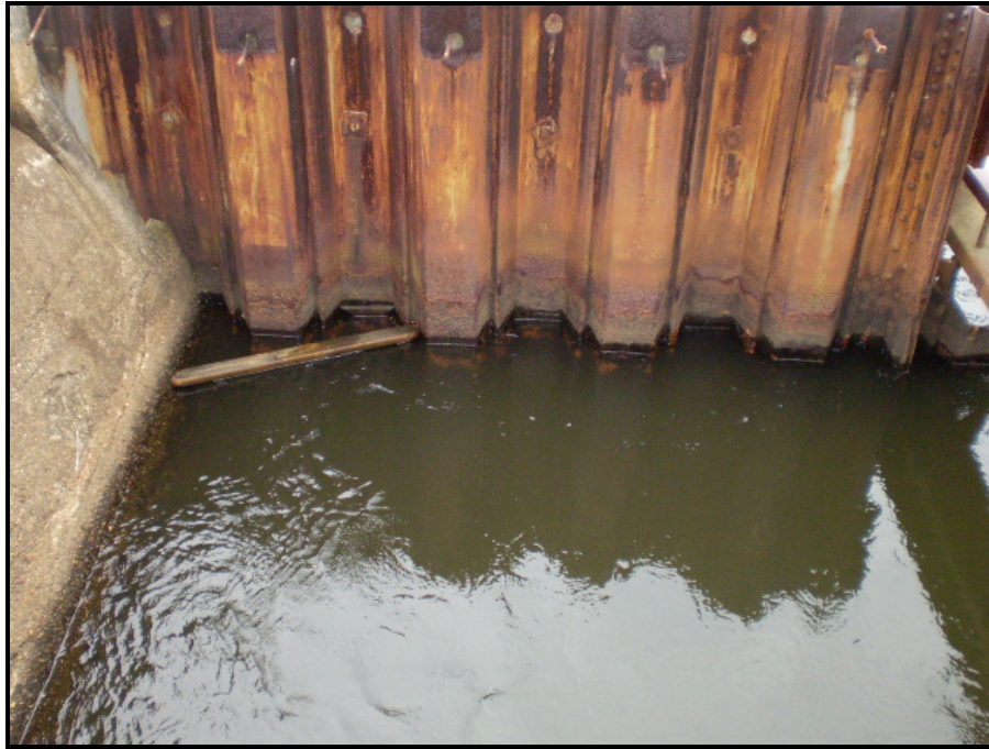
Photo 11 West Elevation of East Steel Sheet Pile Weir Wall
