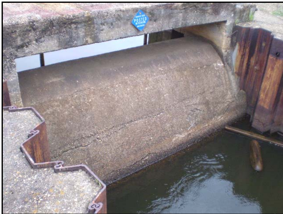
Photo 10 South Elevation of Concrete Weir Wall (Note Scale Throughout)
