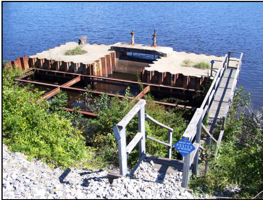
Photo 5 South Elevation of Weir (Looking Northwest)
