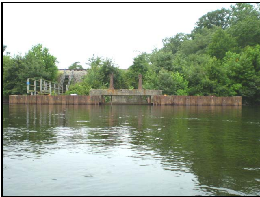
Photo 6 North Elevation of Weir
