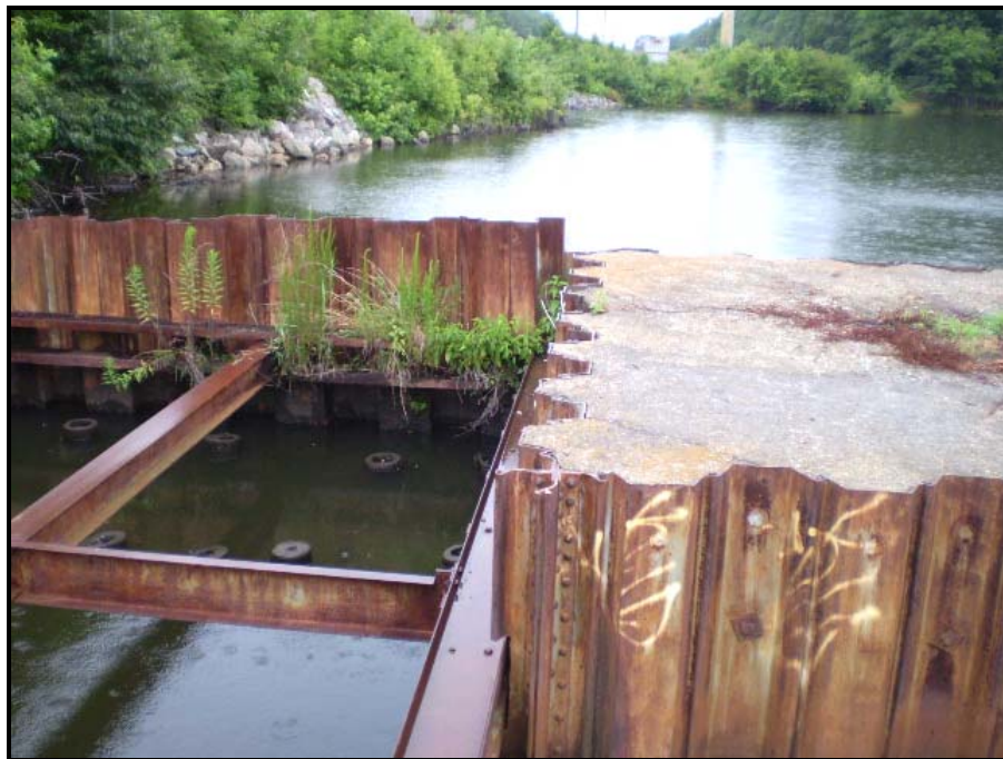
Photo 14 Looking West into the Weir Showing Timber Piles Within Weir
