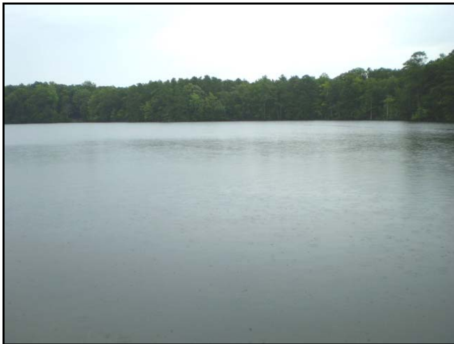
Photo 4 Looking South (Downstream)
