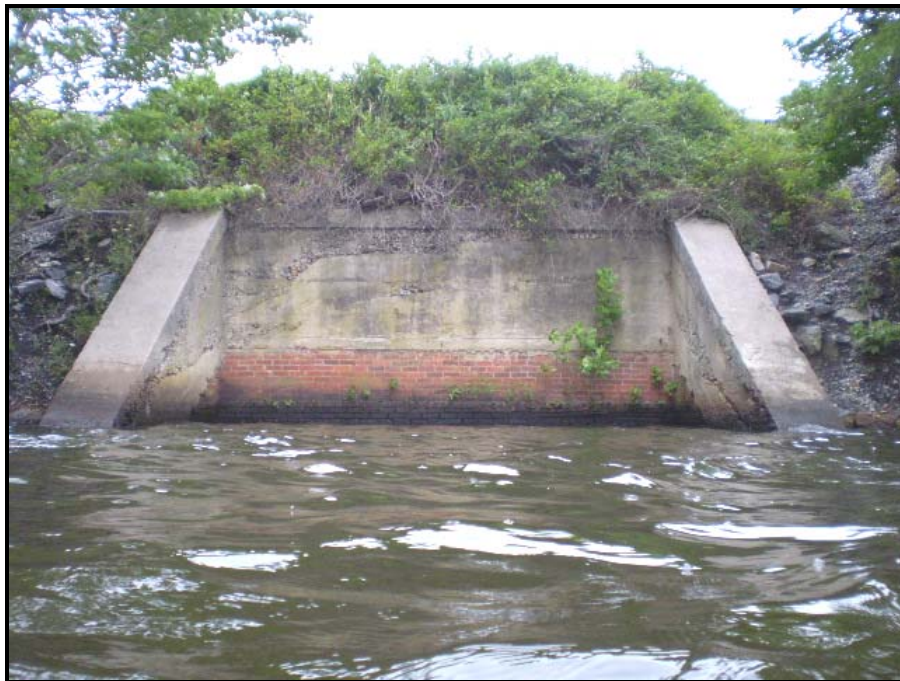
Photo 2 South (Downstream) Headwall
