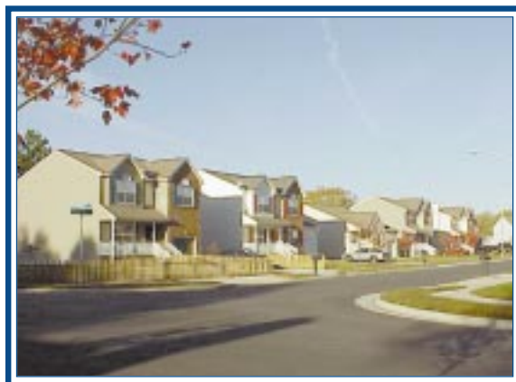
The Villages of Newport on the former Glen Gardens site.
