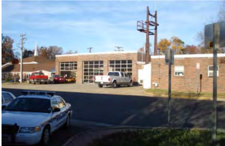
FIGURE 3: FIRE STATION 9 IN DENBIGH
